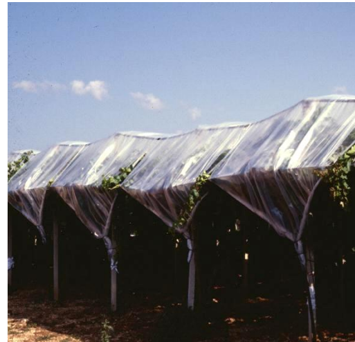
Fig. 4 – “Open” plastic structure for “late covering” table grape vineyard (Apulia region, Southern Italy).
