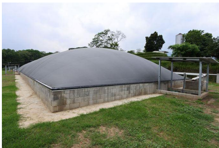
Slika 13. Lagunski digester (Anonymous 1, 2019).
